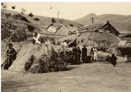
Refugees and refugee sheds at Jiangnan Cement Plant
