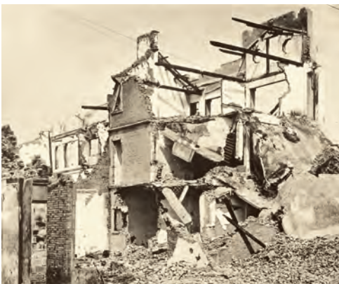
House debris on Taiping Road
